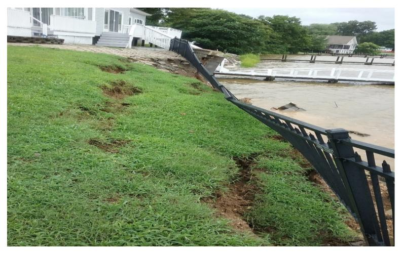
Damage to Property Due to Collapsed Retaining Wall (July 2018)
